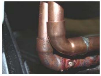
This is a close-up photo of the two elbows in the far left of the picture above. Note that the upper connections are not soldered or brazed – they are to be a slip fit. This will allow the muffler to be removed and re-installed without having to solder the connections.
